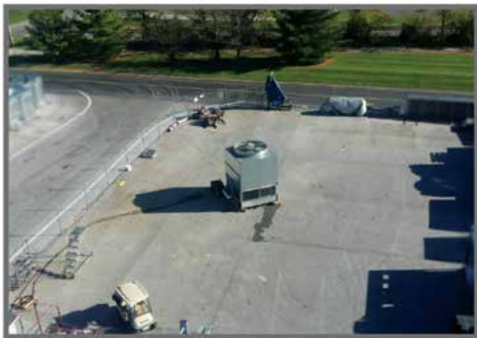
Figure 8: Picture of test site. Condition during Unit 1 test.
